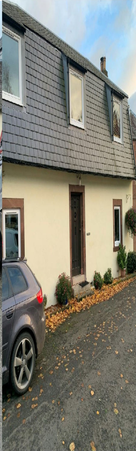
UPVC Tilt & Turn windows installed across the road from Applicants House.
